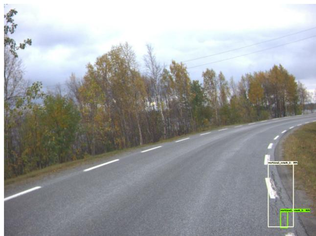
**Figure 17.** Mixed boxes—Model 4. The green box represents the vertical cracks while cyan colored box is the horizontal cracks.
