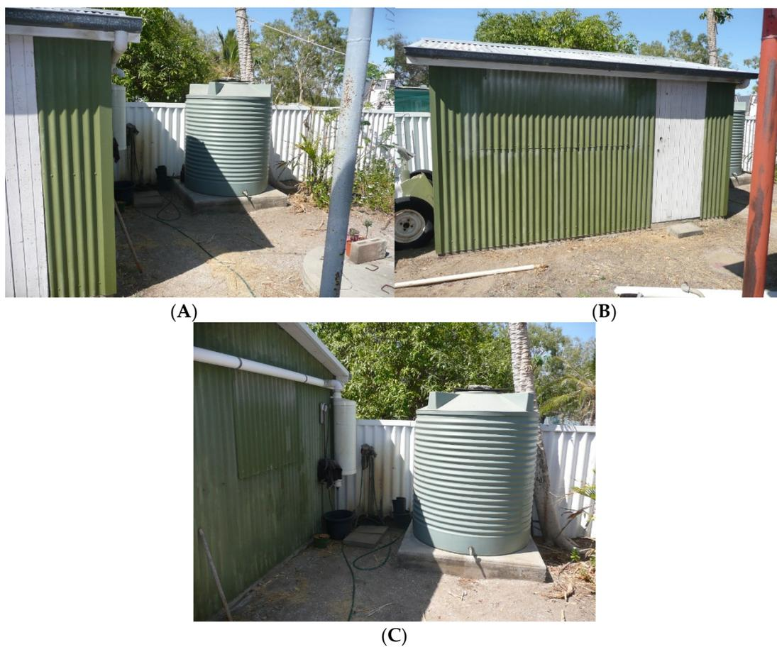
**Figure S4.** 12 Riverview Drive Karumba. (A) PVC tank; (B) Colorbond roof; (C) PVC downpipes and tank.
