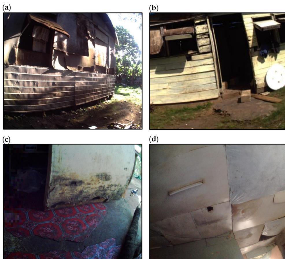
**Figure S2.** Structural damage and building quality of housing stock: (a) House constructed from metal sheet and patched up with lumber, cardboard and fabric; (b) House with damaged window structures and insufficient natural lighting inside; (c) Evidence of rotten wood and water damage to door frame; (d) Ceiling with evidence of water damage and ceiling tiles missing or replaced with plastic sheets.
