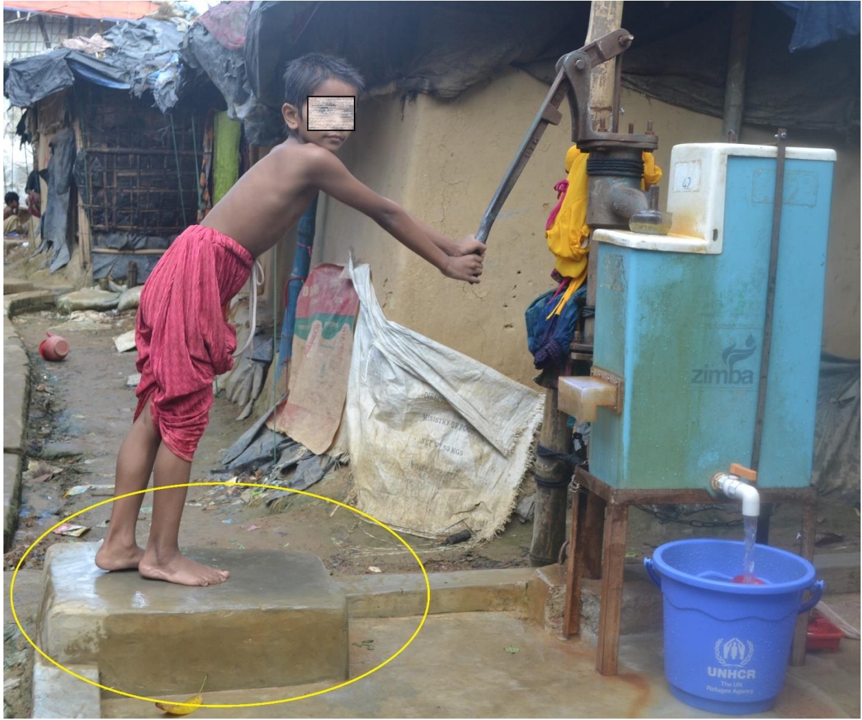
Figure S3. Raised footstep to resolve the increased height of tubewell after Zimba installation, Rohingya camp, Cox's Bazar-2017.
