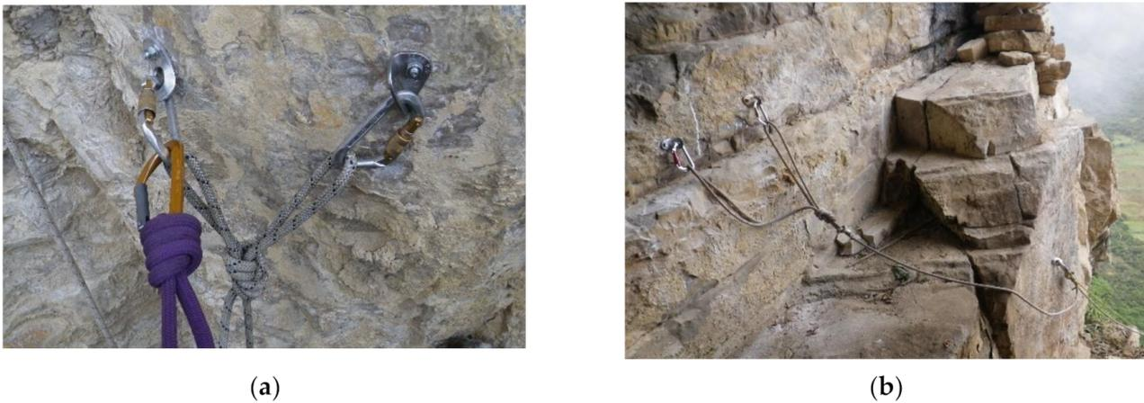
**Figure 11.** (a) Anchor system rigging with a double figure of 8 on the bight (called also bunny knot or bunny ears); (b) in-line anchor system, right anchor supports all the load and left anchor only goes into the load in the case of right anchor failure.
