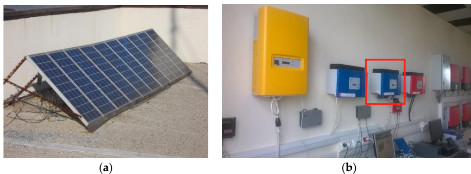
Figure 4. The components of the subsystem 1: (a) 10 photovoltaic panels; and (b) the Sunny Boy SB2100TL inverter.
