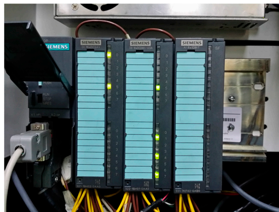
Figure 9. Programmer logic controller (PLC).
