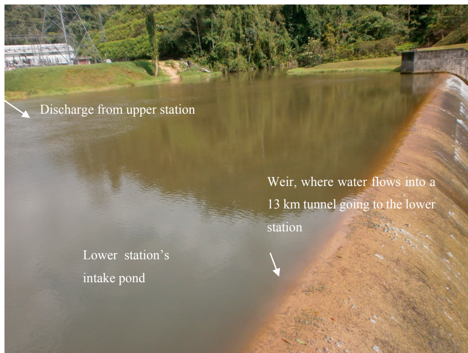
Figure 2. Lower hydroelectric intake pond with spillage.
