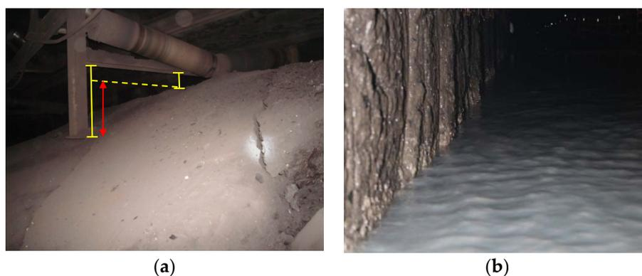
**Figure 2.** Field floor heave of gob-backfilled GER. (a) Floor heave affects the roadway transportation; and (b) floor water inrush.
