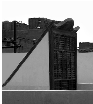
Figure 2. A traditional wind tower in Cairo, Egypt [21].
