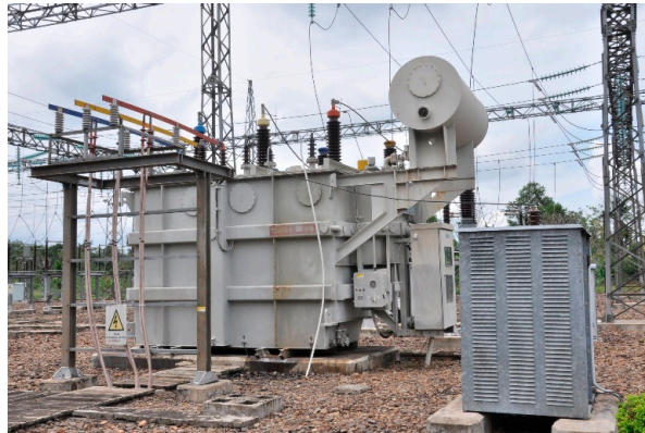
Figure 1. Example of 150/20 kV transformer with a capacity of 60 MVA.
