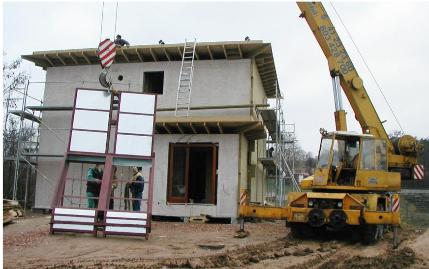
**Figure 8.** Installation of an experimental solar chimney on the roof of a demonstration house with a hybrid ventilation system.
