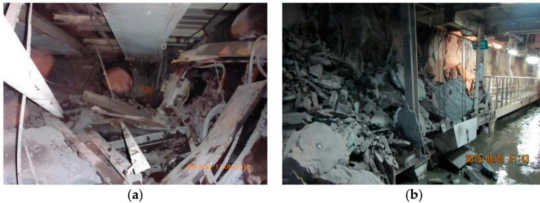
**Figure 5.** Rockburst damage from the 31 May 2015 event.
