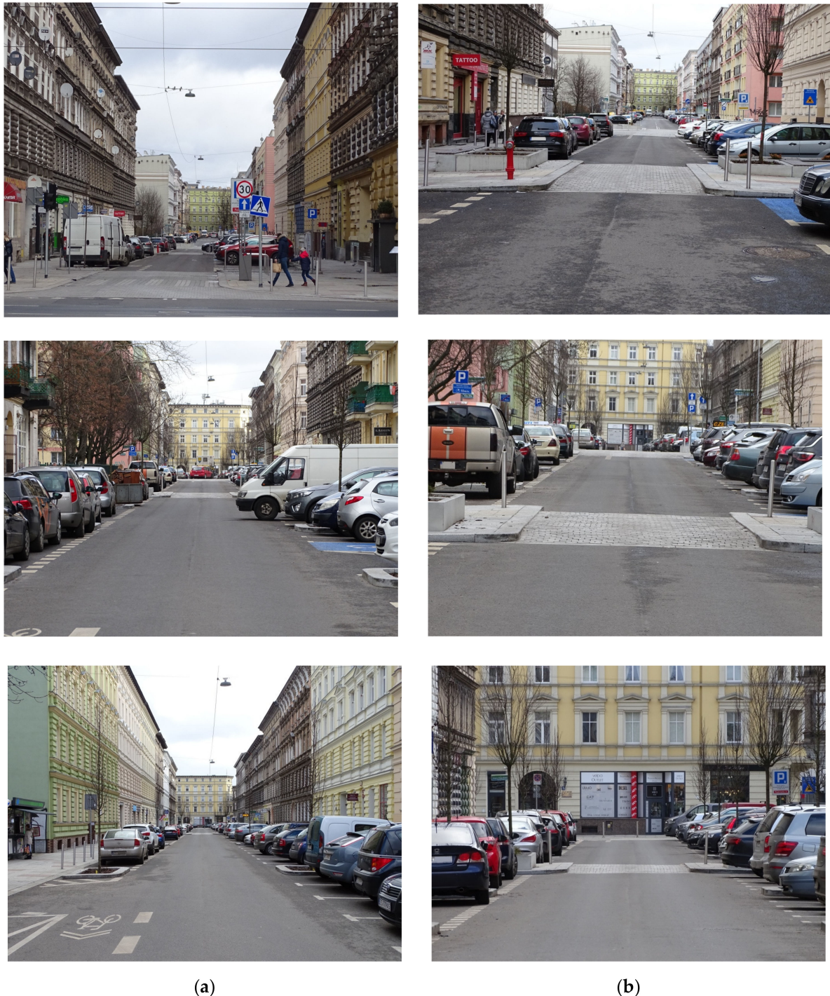
Figure 5. Test sections before and after chokers with raised pedestrian crossings in testing ground No. 1, No. 2 and No. 3: (a) test section before choker; (b) test section after choker. Source: own work of the author.
