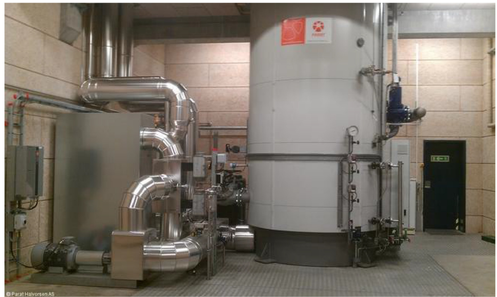
Figure 13. Example of an installed 10 MW electrode boiler from Parat in Denmark.
