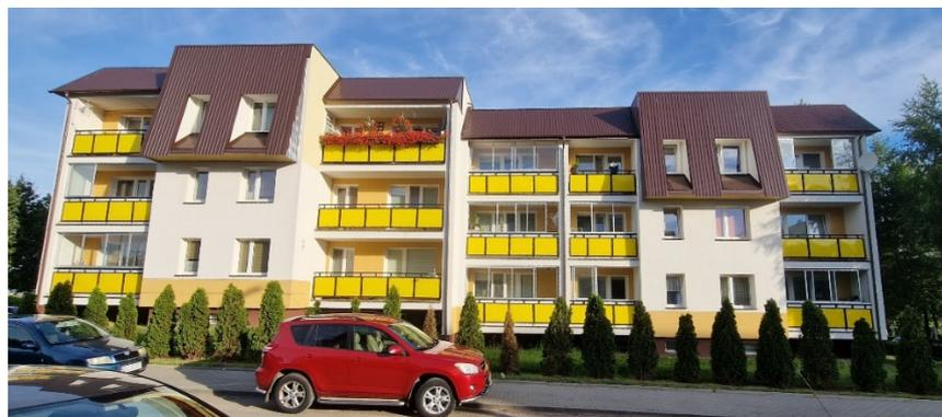
**Figure 2.** View of a typical building (B3) adopted for the study, made with large-block prefabricated CŻ technology, 3-story, 2-cage [photo taken by authors].
