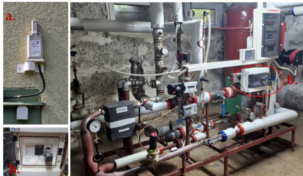
**Figure 4.** Egain Hub weather forecast receiver (a) mounted on the outside wall of the building and the signal transmitter (b) mounted on the heating substation [photo taken by authors].
