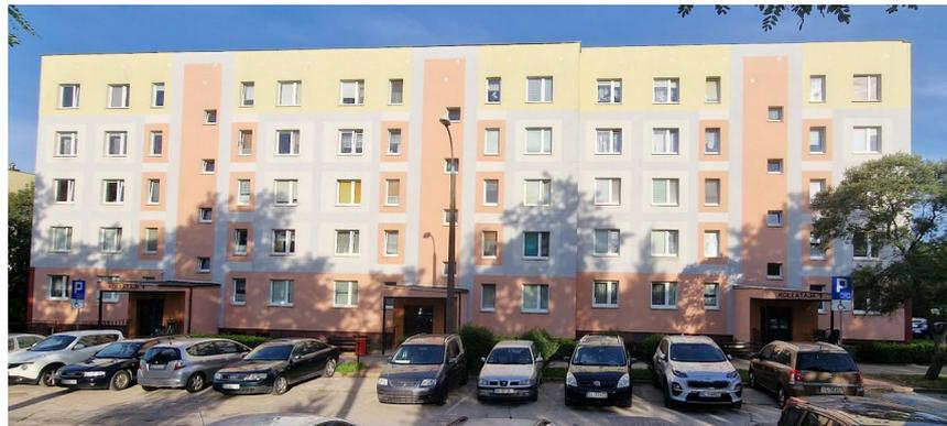
**Figure 1.** View of a typical building (B19) accepted for the study, made with OWT -67N large-panel prefabricated technology, 5-story, 3-cage [photo taken by authors].
