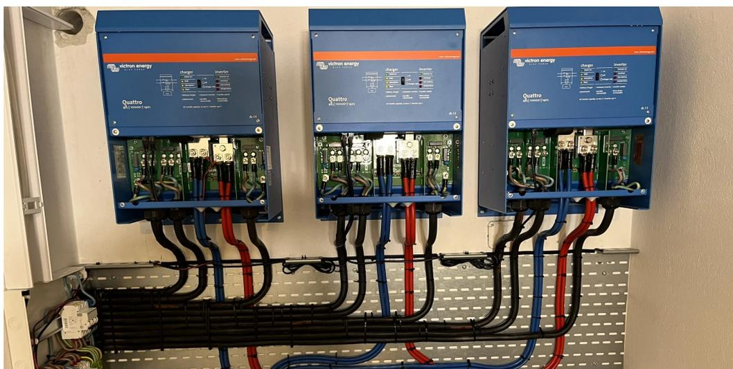
**Figure 3.** Triple Victron Quattro inverters (source <https://enerp.pl/project/victron-ess-kamienica-30kva-404kwh>), accessed on 2 January 2023.
