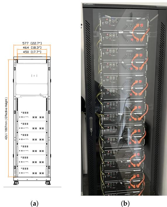
**Figure 4.** Example of batteries and inverter installation: (a) one-phase installation including 1 inverter and 6 batteries; (b) separate batteries mounted on a rack (source <https://enerp.pl/project/victron-ess-kalisz-45kva-50kwh>), accessed on 2 January 2023.
