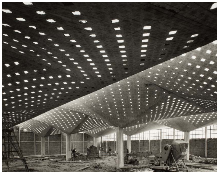
Figure 9. Factory in Mexico under construction with a tilted roof design similar to a saw-tooth profile to allow diffuse lighting into the interior space. (Photo courtesy of Candela Archive, Princeton University).
