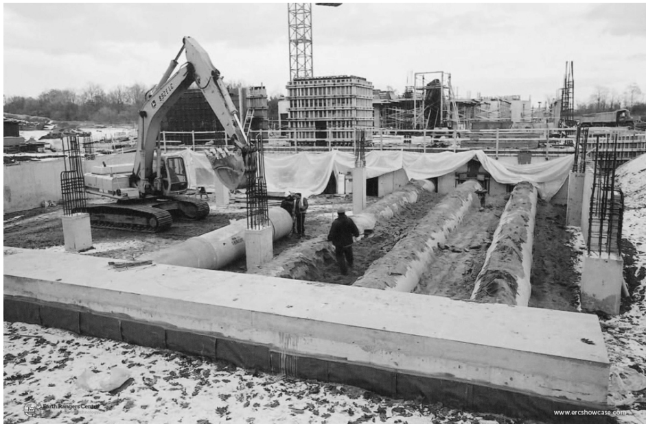
Figure 3. A large diameter earth air heat exchanger under construction. Phot by R. Lay, Enermodal Engineering, by permission.
