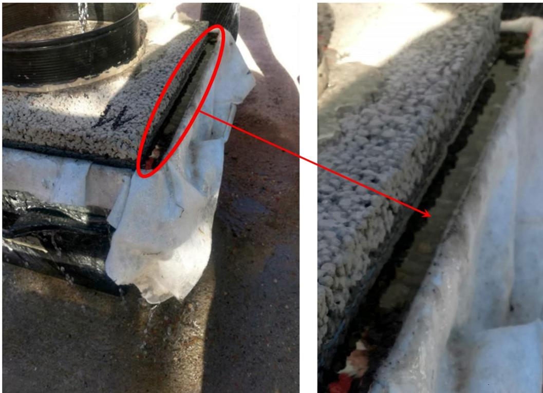
**Figure 9.** Water film as a result of a discrepancy in pervious concrete infiltration and unbound base course (UBC) exfiltration.
