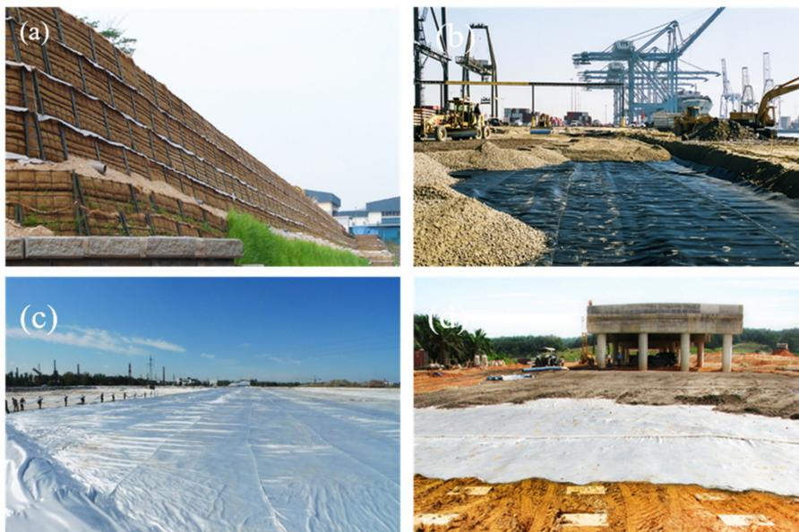
Figure 8. Some applications of geotextile reinforcement: (a) reinforcement of slopes; (b) reinforcement of embankment; (c) reinforcement of soft soil foundation; and (d) reinforcement of load transfer platforms.
