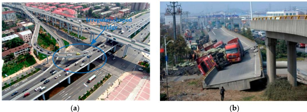
**Figure 1.** Irregularly-shaped bridge. (a) Plan view; and (b) collapse accident.
