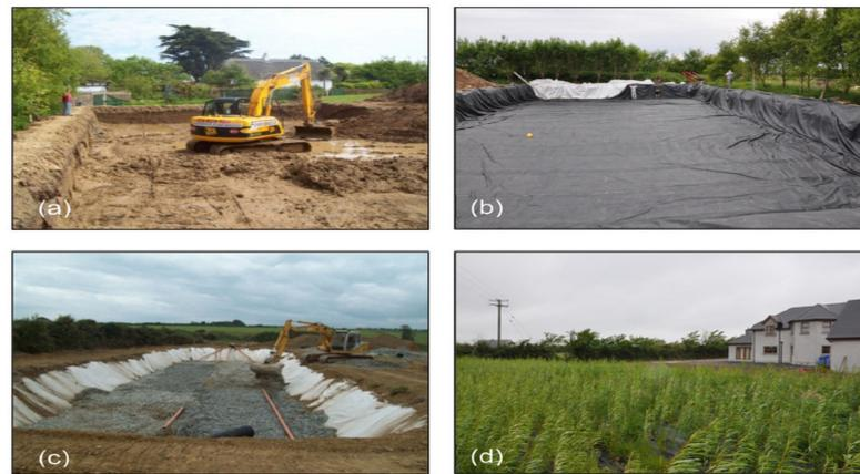
**Figure 3.** Stages in the construction of an evapotranspiration system: (a) excavation of basin (b) laying the impermeable membrane (c) installation of distribution layer, and (d) initial growth of the willows [29].
