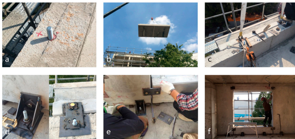
Figure 11. Construction Process of PC-Wall. (a) Perforation and insertion of anchors; (b) Pulling up by crane; (c) Locating the placement position; (d) Fixation by bolting; (e) Assembly of an angle steel; (f) Finishing of joint.
