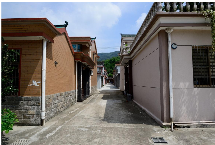
Figure 5. Phase 2 house featuring the brick structure and stone foundation.
