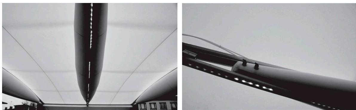
**Figure 6.** Images of the Tensairity® beam used in the Ducati Pavilion.
