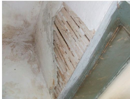
Figure 26. Dividing walls are made of wood and later plastered (Photo: Dušan Tomanović).
