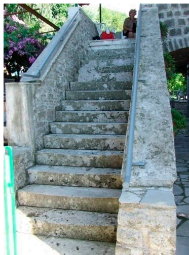
Figure 30. The tread and fence of the external stairway are mostly made of stone (Photo: Dušan Tomanović).
