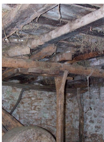
Figure 21. Roof construction is supported by a wooden forked pole (Photo: Dušan Tomanović).
