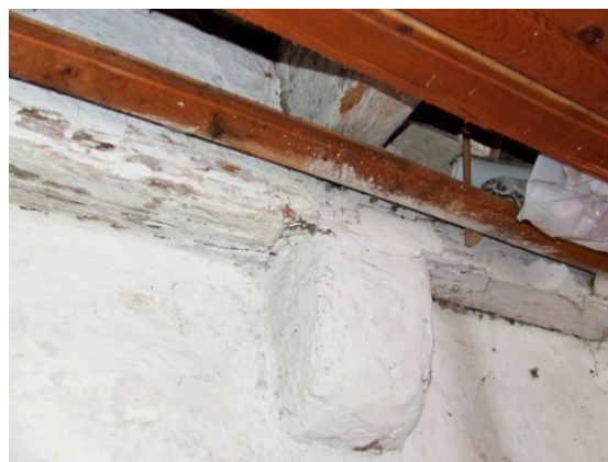
Figure 28. The small bracket carries the floor joist beam on the inner side of the wall (Photo: Dušan Tomanović).
