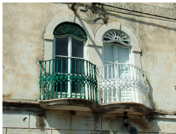
Figure 41. At the beginning of the 20th century, balcony fences were made from wrought iron (Photo: Dušan Tomanović).
