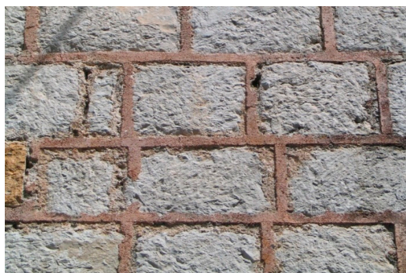
Figure 25. An example of a joint protruding out of the wall lines (Photo: Dušan Tomanović).
