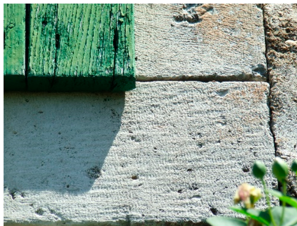
Figure 17. The Korčula stone is soft and easy to process; however, due to its lightness and brittleness, it is rarely used for construction, but only for decorating the facade (Photo: Dušan Tomanović).
