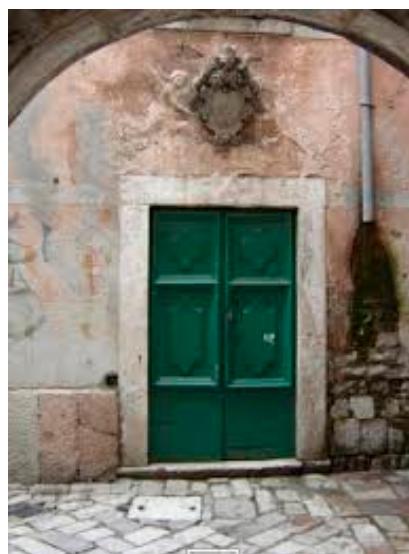
Figure 34. A door with no fanlights is framed with rectangular stone frames (Photo: Dušan Tomanović).
