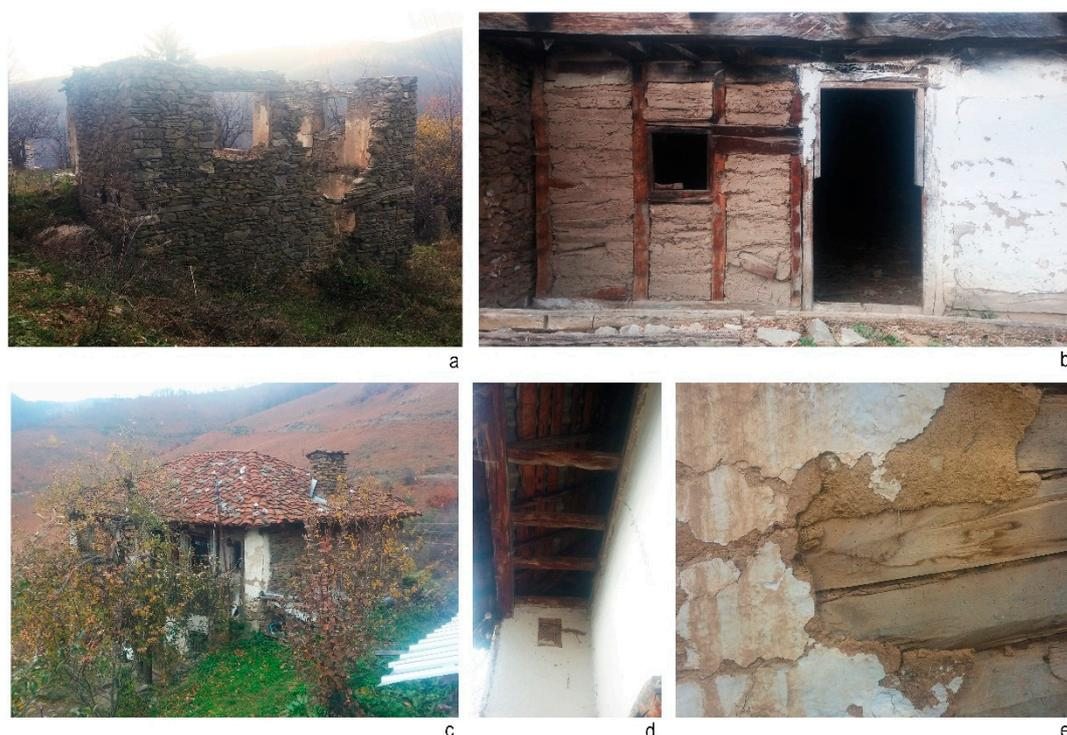
**Figure 10.** Structures and components of Sirinić houses: (a) remains of exterior stone walls of a two-story house; (b) bondruk structure; (c) original *čeramida* roof tiles; (d) roof eave structure; (e) covering of bondruk wall with a mixture of mud and straw.
