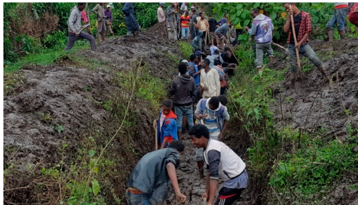
Figure 2. Farmers dredging sediment from a main canal (sediment hotspot section) at Ketar irrigation scheme (August 2017).
