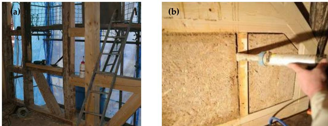
**Figure 7.** (a) Restoration of timber framework (b) TYPHABOARD infill and sealing of joints by typha swelling mortar, pictures: Fritsch Knodt Klug.
