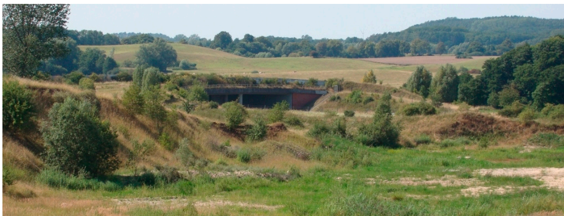
Figure 24. Example of a green bridge located in a rural area, featuring parabolic noise barriers extended by contiguous earthen berms.
