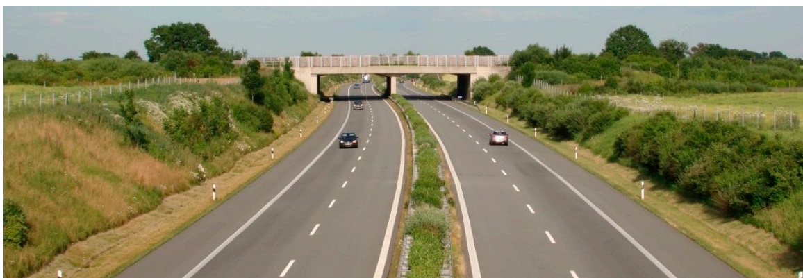
Figure 13. Plantings of different species and heights provided on the road cutting slopes.
