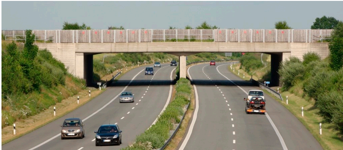
Figure 12. Central recess in a wooden noise barrier located over the median strip.
