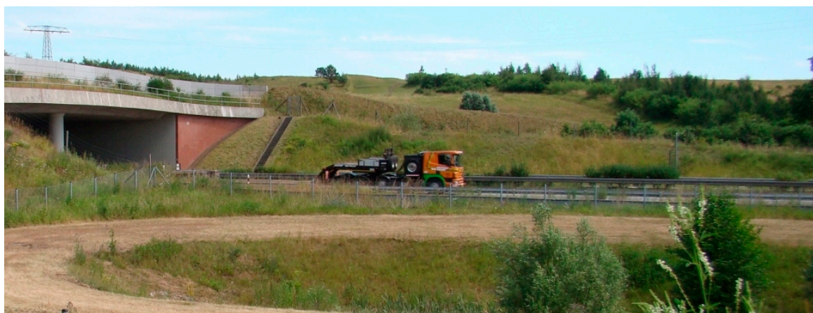
Figure 25. Example of a contiguous, tight connection between the noise barrier and earthen berms.
