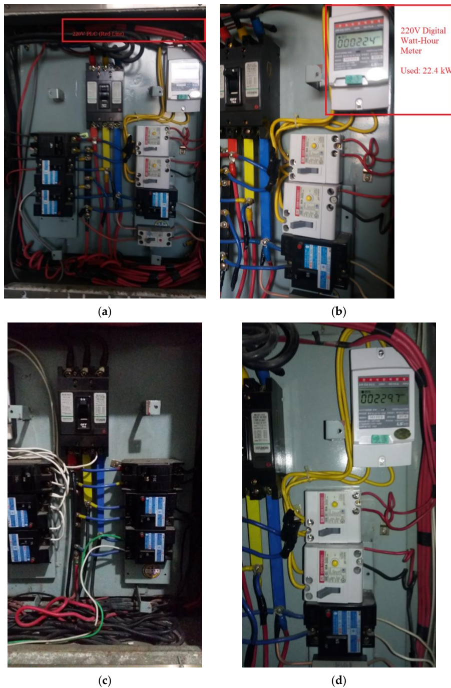
Figure 19. PLC System and Digital Watt-Hour Meter installed in an old home environment. (a) PLC Centric Monitoring System (Main part); (b) Digital Watt-Hour Meter; (c) Before Installation (PLC and Digital Watt-Hour Meter); (d) Digital Watt-Hour Meter (1 July 2018–30 June 2019).
