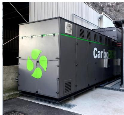
**Figure 1.** C-700—HTC plant, Carborem, fully operative at a waste water treatment plant.
