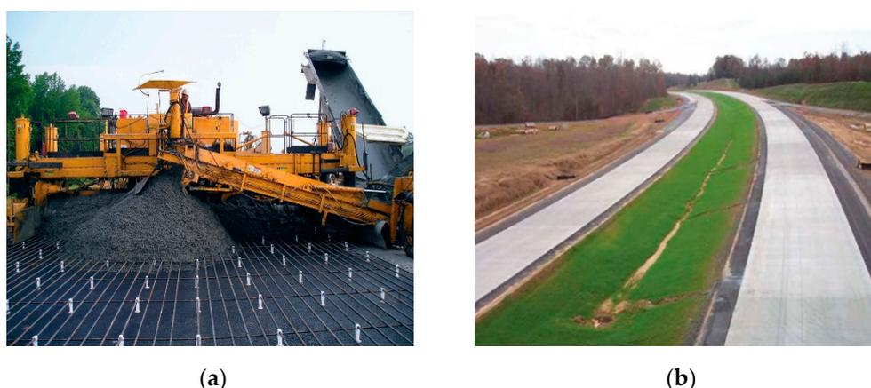
**Figure 1.** (a) Continuously reinforced concrete pavements, (b) during construction and after construction [2].
