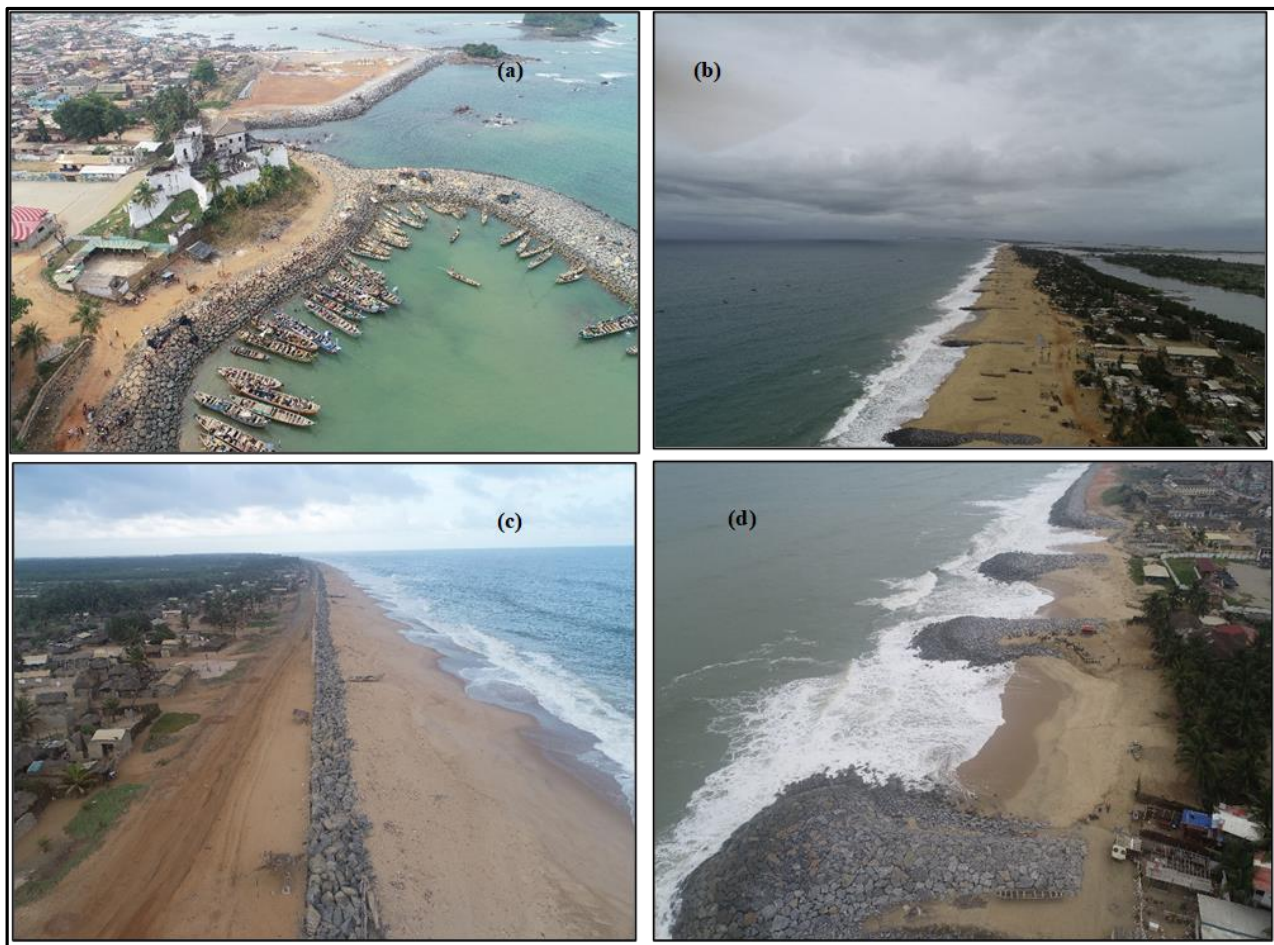
Figure 11. Coastal infrastructure along the coast of Ghana showing (a) Axim sea defence; (b) Blekusu groyne field; (c) Atokor revetment; and (d) Cape Coast (Oasis Beach) groyne field and seawall, all implemented using the HTL and grey infrastructure [55].
