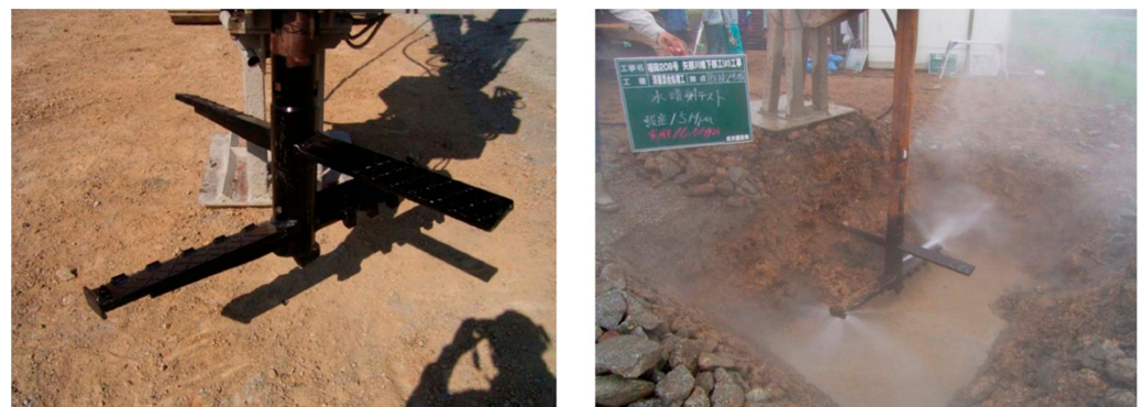
Figure 4. Water spraying demonstration by MITS monitor.
