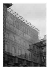
There are also facade and roof systems where aluminium is used in window and glazing frames and glazing spacers. The function of these systems is to provide daylight, visual contact between the exterior and the interior, provide protection against the weather (rain and wind), provide passive solar heating gains, help keep interior thermal comfort, and keep the energy use for operation at a minimum.
