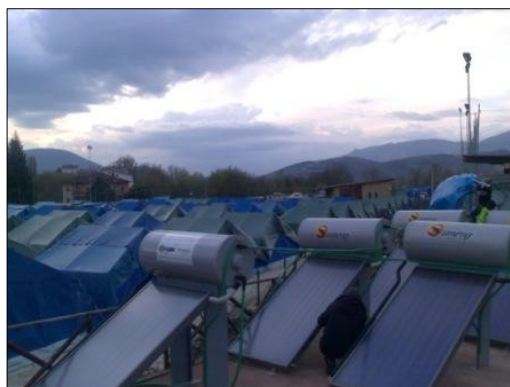
Figure 5. Integrated collector-storage systems (ICS) Solar thermal plant in Lilletta camp.
