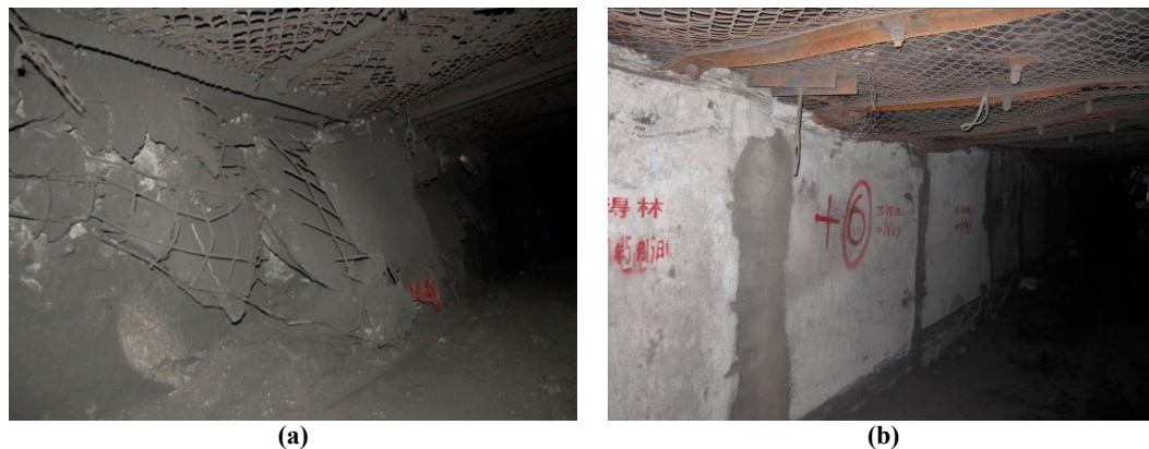
Figure 19. Profile of the RGSG under hard roof: (a) before roof pre-split; and (b) after roof pre-split.
