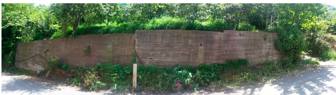
Figure 10. Very limited wall vegetation on a smooth concrete wall surface.
