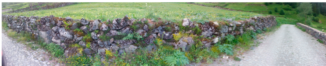
Figure 12. Wall vegetation (the main material is permeable at the crest).
