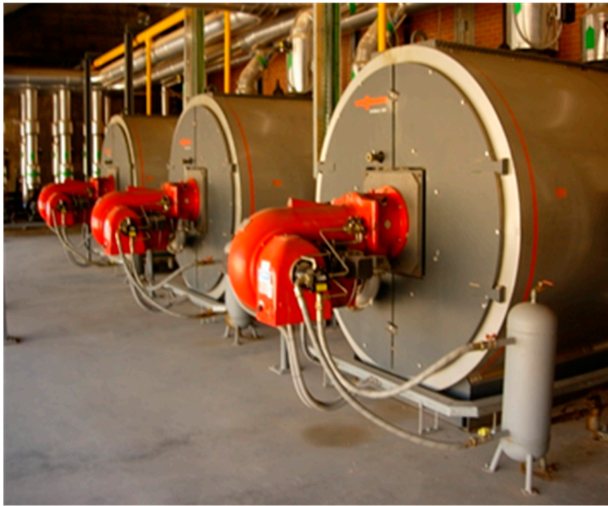
Figure 2. Set of boilers with 3200 kW nominal power.
