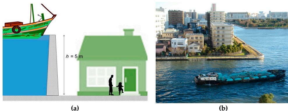
Figure 10. (a) Illustration showing a sinking coastal community protected by a 5-meter thin dyke, such as the ones currently used in Jakarta; (b) Robust coastal dyke defending Koto ward in Tokyo (note that the houses on the left are a few meters below sea level).
