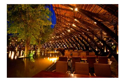
Figure 2. Bamboo used as structural elements in Vietnam (Architect: T.-N. Vo).
