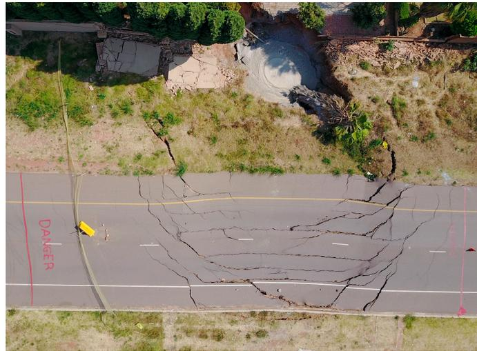
**Figure 3.** A sinkhole, and associated tension cracks, that resulted in road closure in Gauteng, South Africa in 2018. The sinkhole is in the process of being rehabilitated and has been filled with concrete. (photo credit: Dilnaaz Patel).
