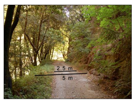
**Figure 2.** Little Creek road with dimensions, note the steep cut- and fill-slopes.
