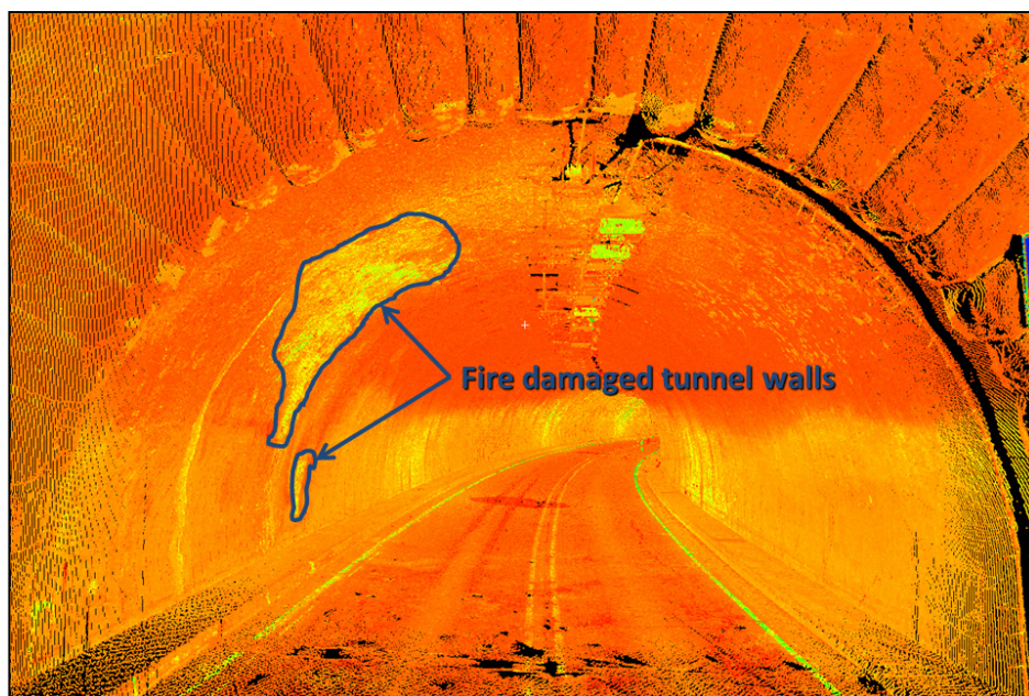
Figure 12. Close examination of the intensity shaded point cloud (static scan) shows additional, minor damage to concrete in a tunnel in Oregon (Courtesy of Oregon DOT).
