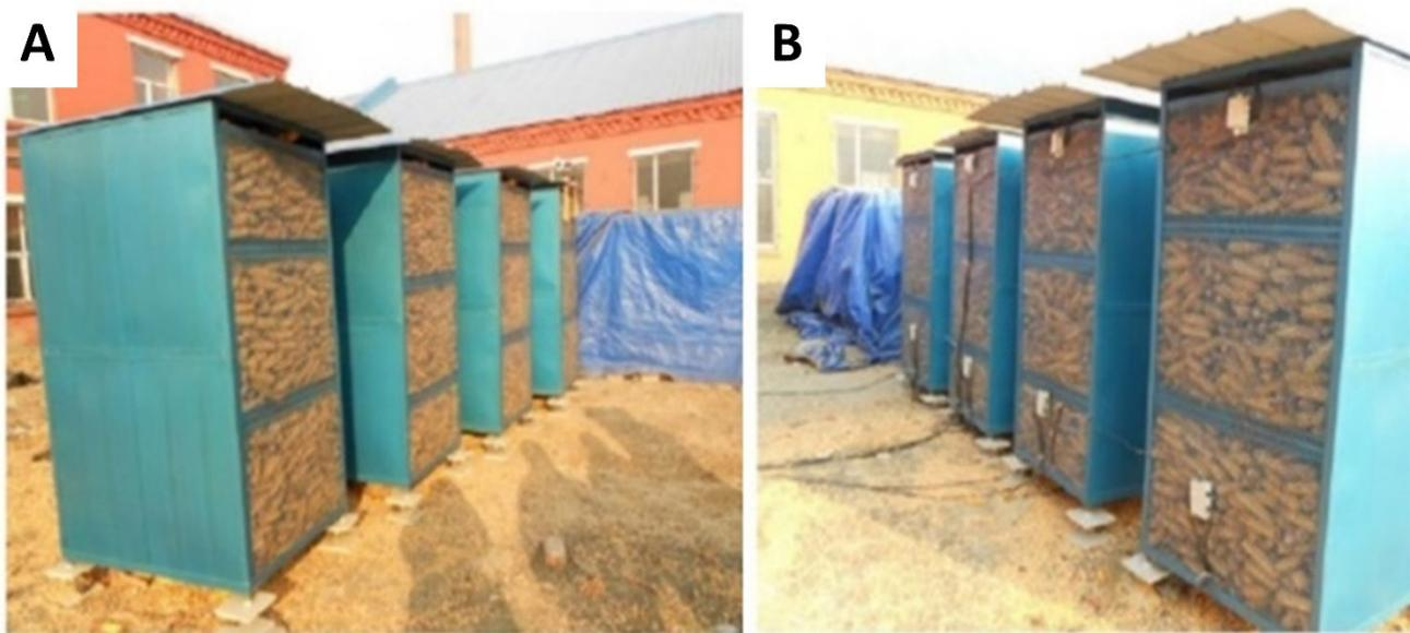
**Figure 6.** Natural ventilation corn ear storage silos. (A) Rectungular steel mesh facing east; (B) Rectungular steel mesh facing west.
