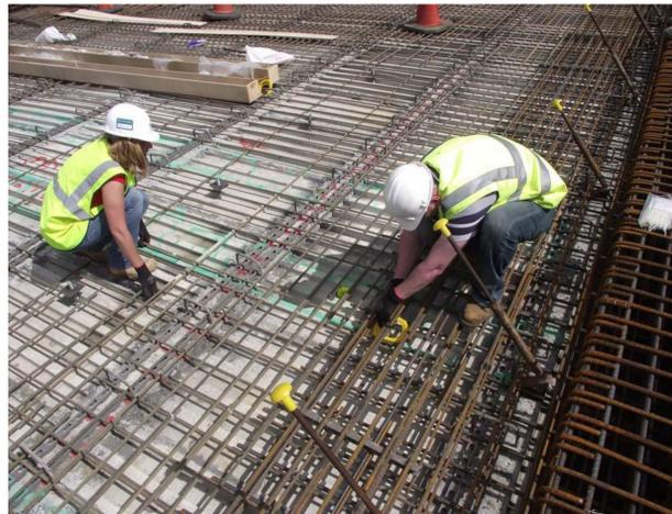
**Figure 5.** Positioning of the fiber bragg gratings (FBG) sensors.
