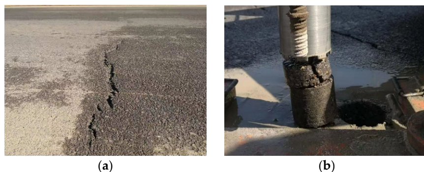
Figure 1. Interlayer slippage of PU mixture composite pavement. (a) Interlaminar slippage. (b) Interlaminar shedding.
