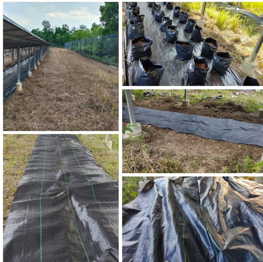
Figure 9. High-quality weed mats have been used as weed control measures directly under solar PV arrays for further crop cultivation.
