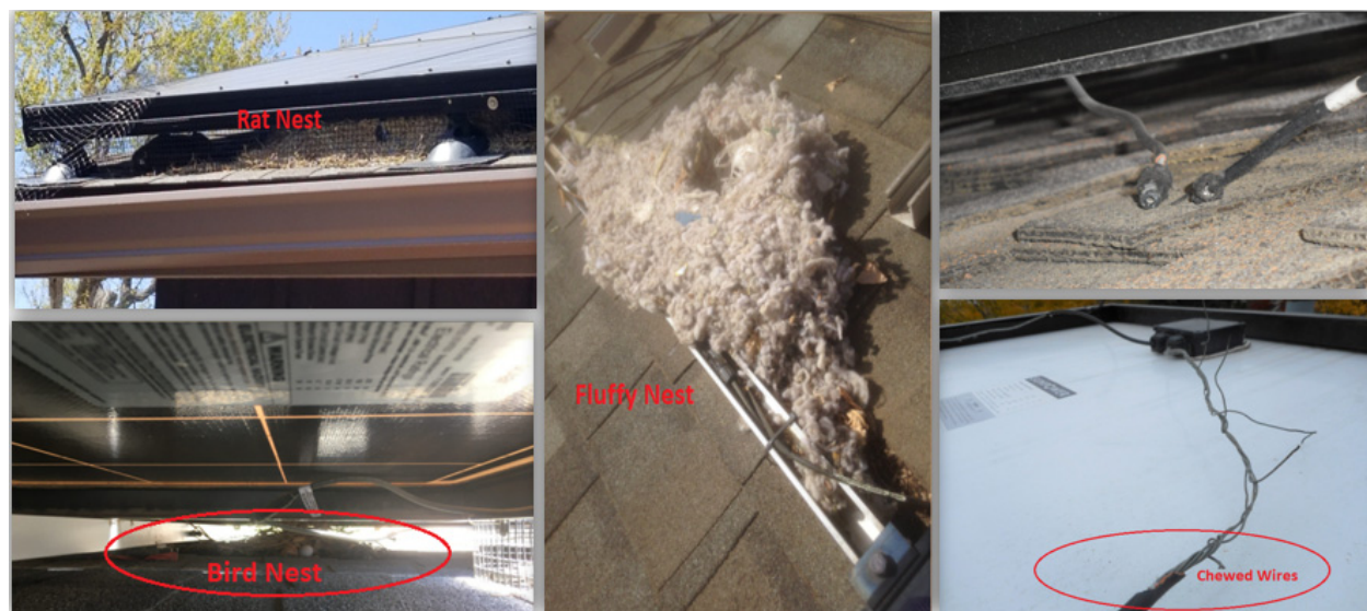
Figure 3. Pest damage to solar PV arrays [25].
