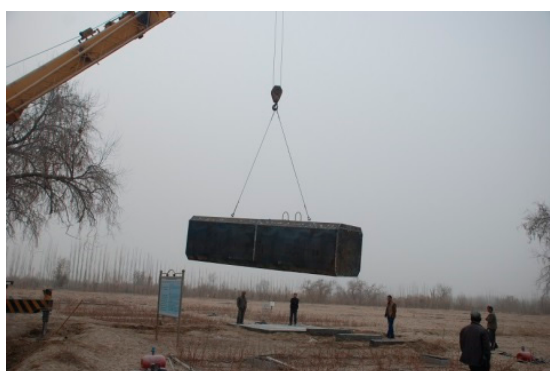
(a) installation of the sedimentation tank
